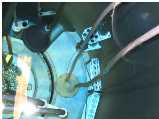
Figure 4. Top view of the reactor core with PE container. A 6 m water column protects people against radiation.
