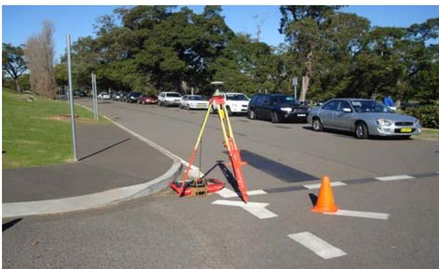
Figure 1. GCP Surveying using GPS
