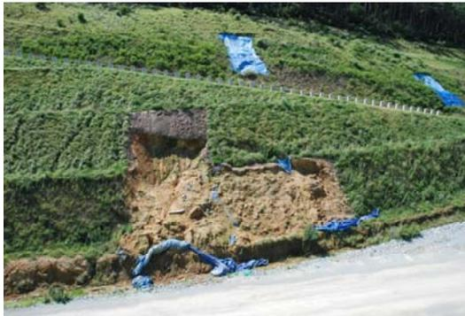
Figure 4. Road Cut and Failure Slope
