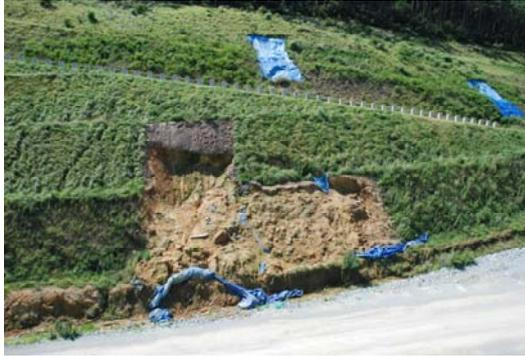
Figure 4. Road Cut and Failure Slope
