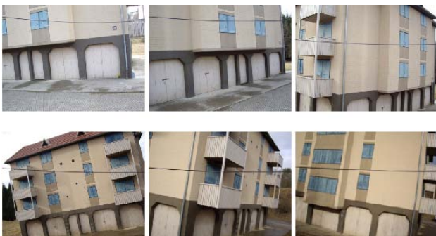
Figure 2. Image sequence Three Walls, images 3, 9, 12, 20, 25, and 28 - Please note the dark approximately horizontal line which stems from the ring around the UAV to secure its rotors against hitting other objects.
