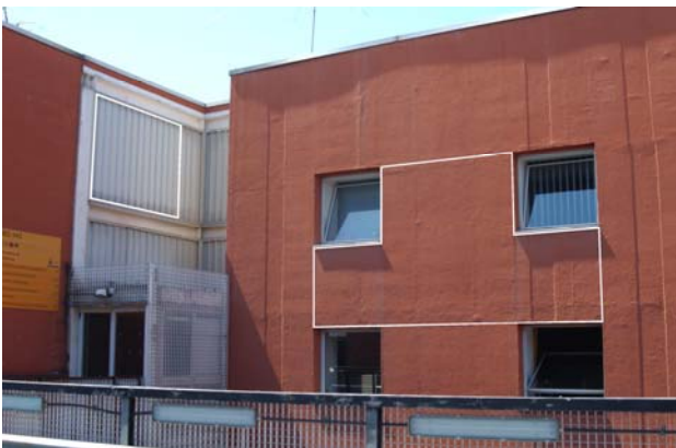
Figure 8. A different view of the building of figure 7
