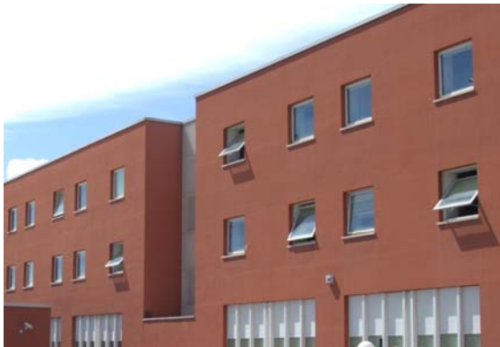
Figure 1. The Land Planning Dept. facade
