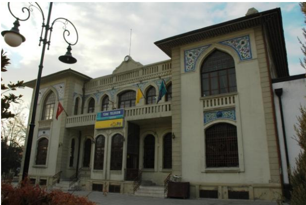
Photo 1. Front façade of the building.
