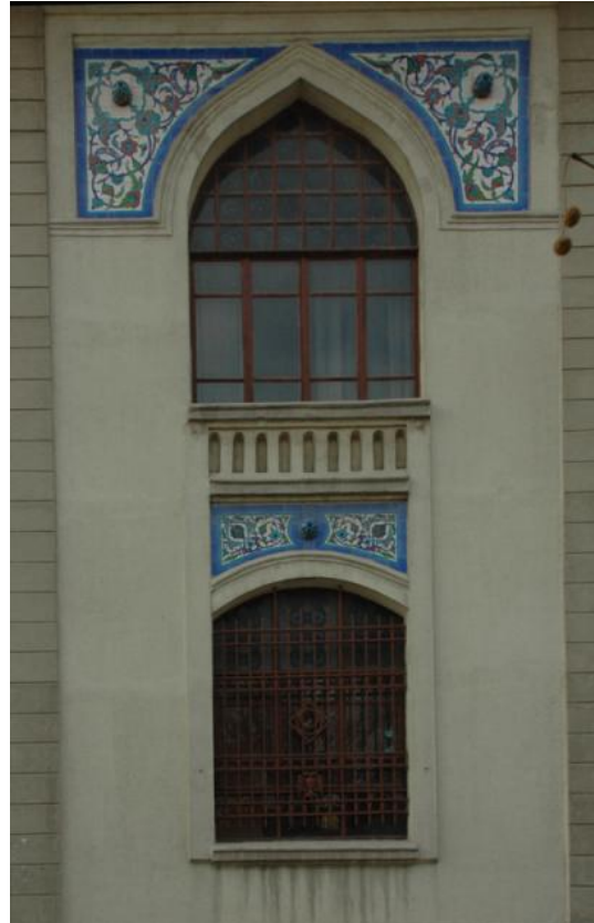
Photo 7. Orthophoto of the façade with tile
