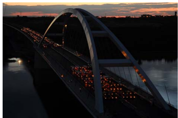
Figure 1. Load test of the bridge
