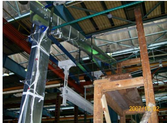
Figure 7. The portal frame equipped with the measurement devices
