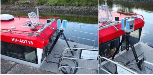
Figure 5: Installation of the terrestrial laser scanner Z+F IMAGER 5006i on a tight mounted tripod on board of the "Level-A".
