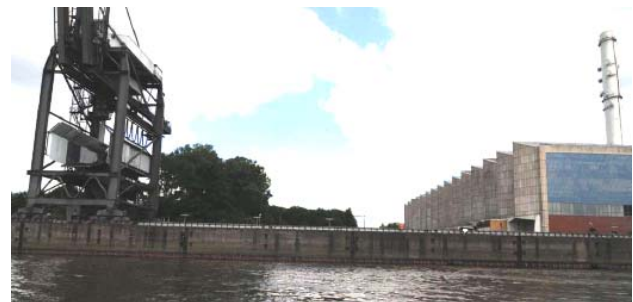
Figure 4: Partial view of the power station in Wedel with embarking crane (left) and factory hangar (right).
