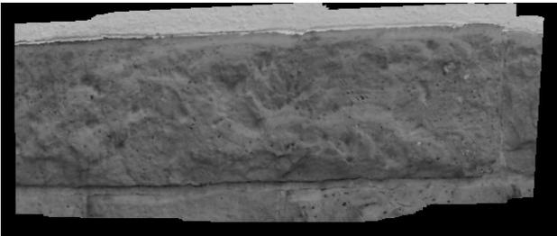
Figure 5. Rectified panorama patch using homography decomposition following [3]
