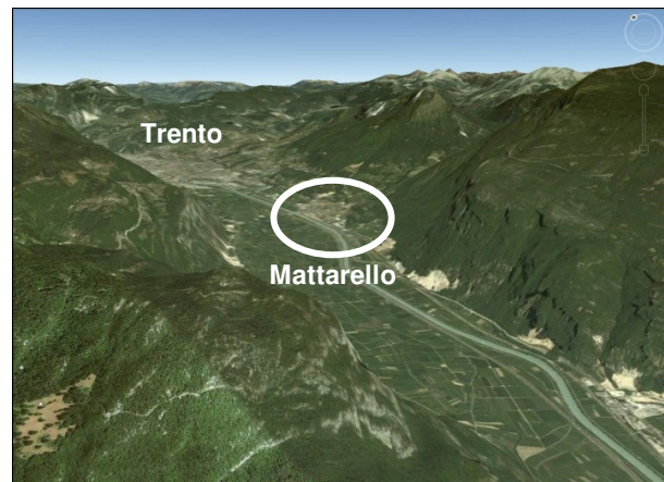
Figure 1 – Aerial view (Google Earth) of the Adige valley in the Alps, with the location of the test site: Mattarello, Trento, Italy.
