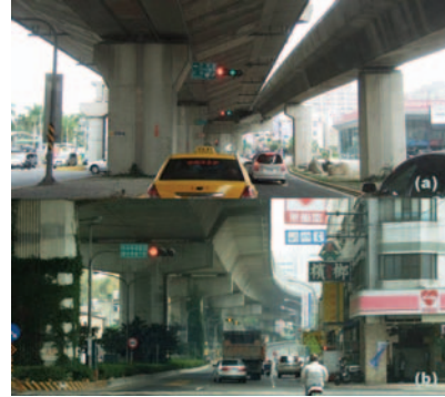
Figure 5. Typical views in the first field test in Kaohsiung
