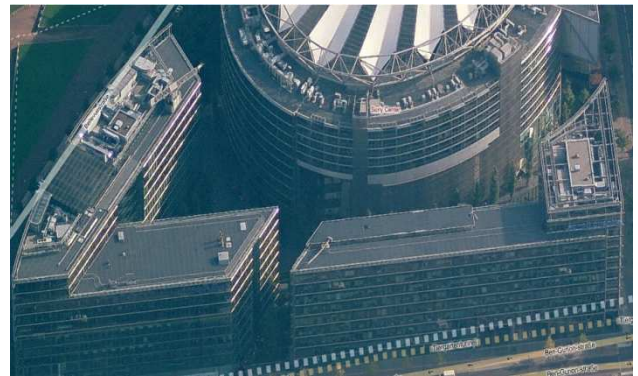
Figure 6. Oblique view aerial image
