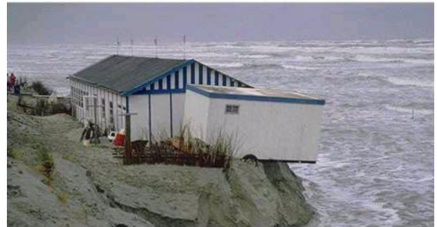
Figure 1: A real example of a dune erosion on the Dutch coast and the possible consequence [GoogleEarth].
