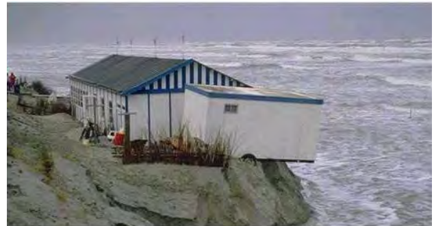
Figure 1: A real example of a dune erosion on the Dutch coast and the possible consequence [GoogleEarth].
