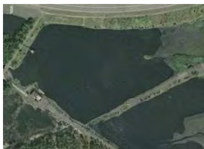
Figure 6. Final sedimentation pond in an aerial photo from 2003
