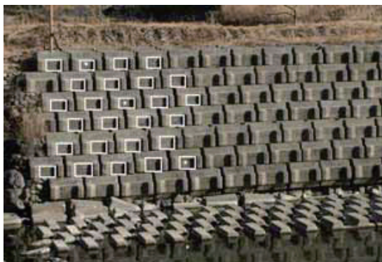
Figure 1.1. Shore-protection blocks and test surface
