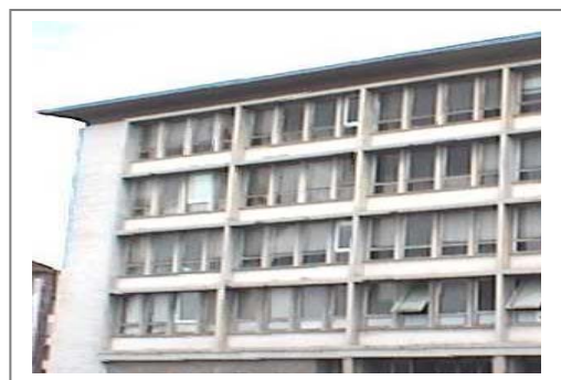
Figure 1. Photograph of the building under study
