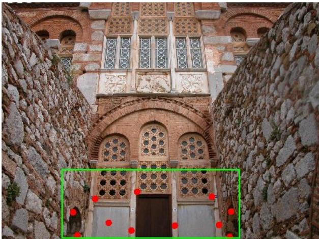
Figure 6: Finally accepted control points (2<sup>nd</sup> scan)
