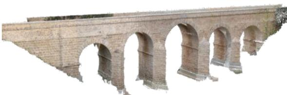
Figure 3. Global point cloud of the Segura Bridge.
